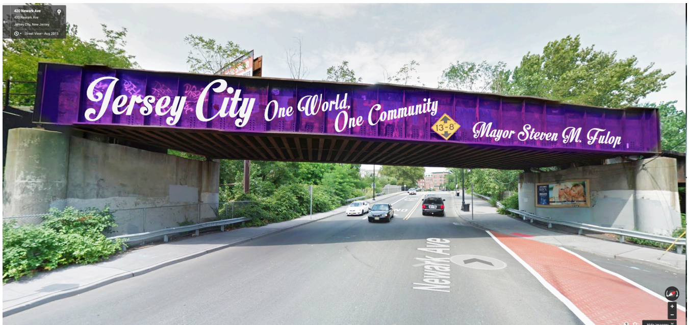
Grand Street Trestle
